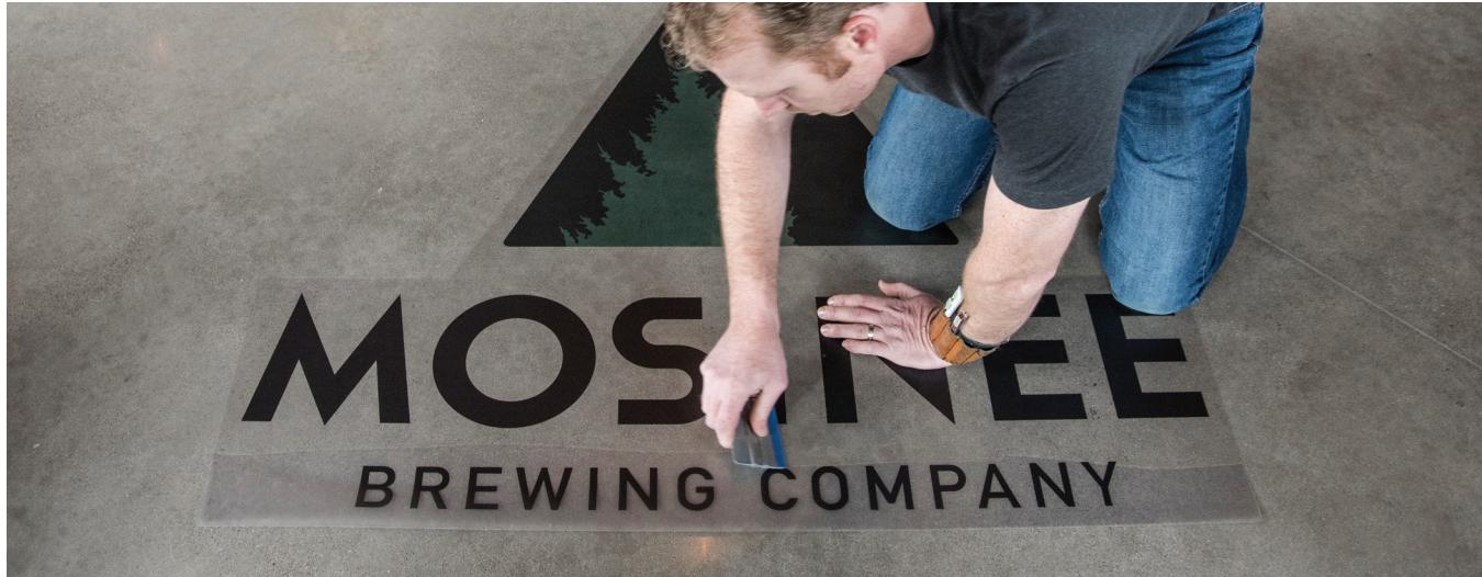
The Walk-On Graphics® two part system includes a printable vinyl base film and a UL 410 slip resistant overlaminates to create durable floor signage applications.
